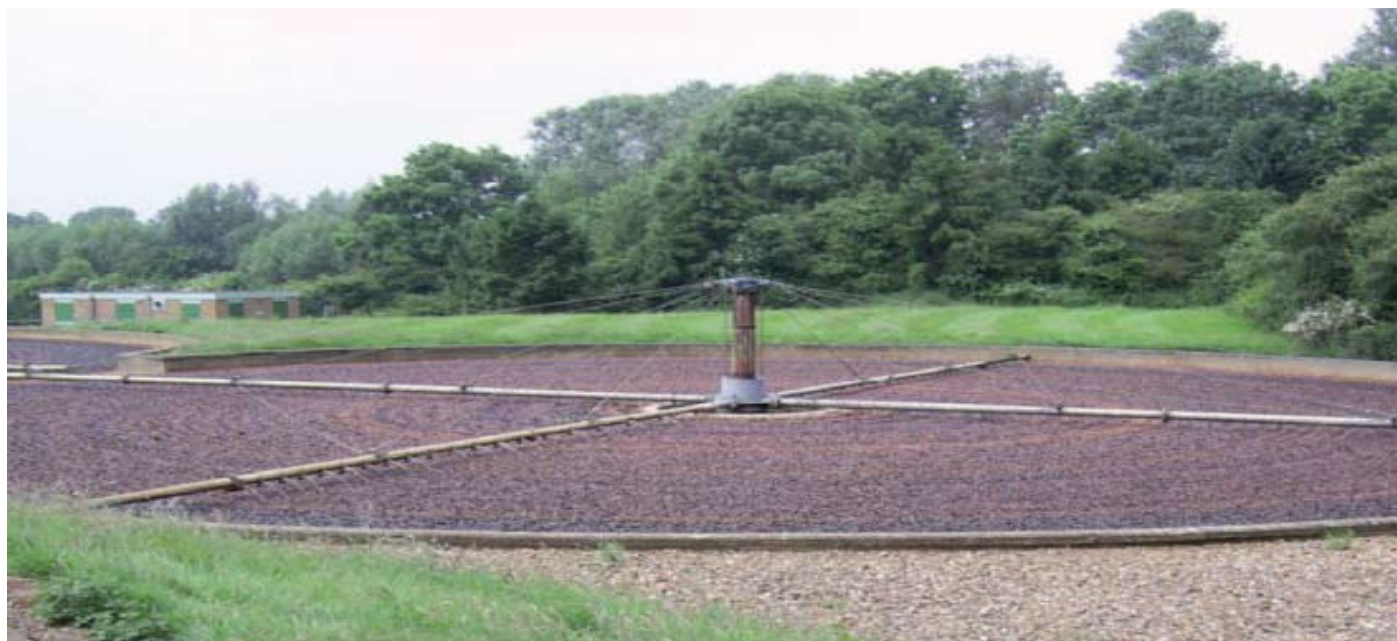
Customer's water treatment facility
